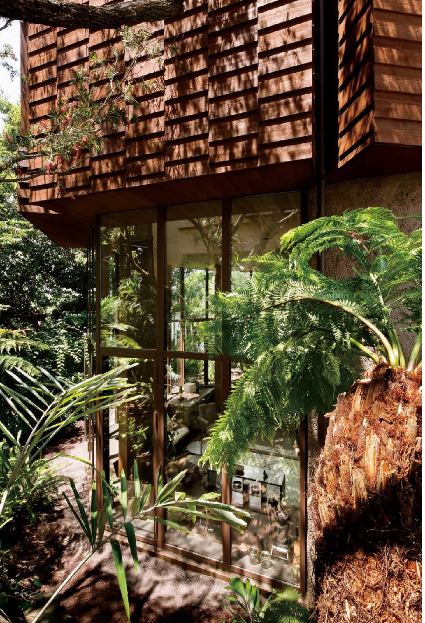
Todoroki House in Valley / Tane Tsuyoshi
