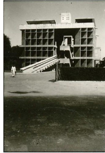
[10] Mill Owners' Association Building (design by Le Corbusier; Ahmedabad, India, 1956). 1957. © Kenzo Tange. Tange made a stop in India on his return from the São Paulo Biennial to study Le Corbusier's buildings.
