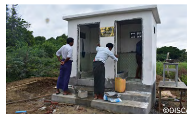
Toilet construction in Myanmar (OISCA JAPAN)
