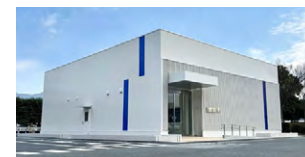
Building housing hydrogen generation device (external view)
