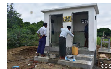
Toilet construction in Myanmar (OISCA JAPAN)
