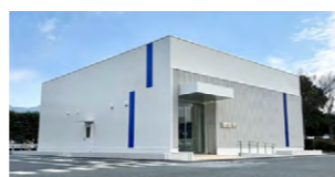
Building housing hydrogen generation device (external view)
