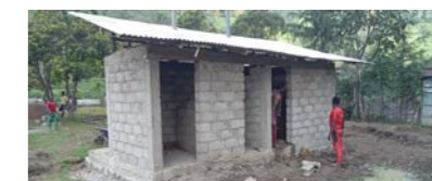
Construction of school toilets in Ethiopia (HOPE International Development Agency Japan)
