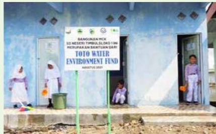
New toilet facility at Timbulsloko First Elementary School, which had suffered from flood damage (Demak Regency, Indonesia)
