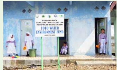
New toilet facility at Timbulsloko First Elementary School, which had suffered from flood damage (Demak Regency, Indonesia)
