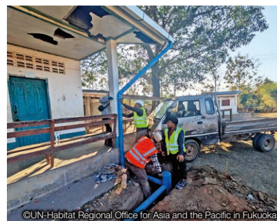
Installation of underground piping
