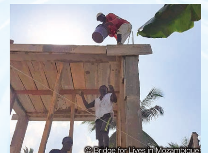
Constructing the water tower © Bridge for Lives in Mozambique
