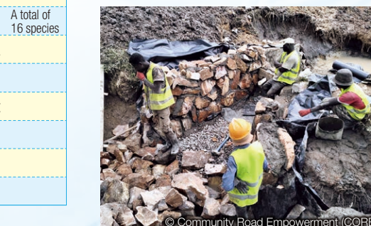
Protection and development of the spring
