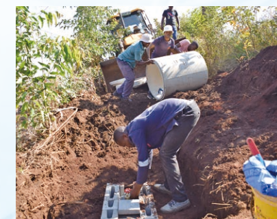
Construction work for pipe network and feedwater systems
